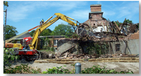
Demolition of Building No. 123 - Kitchen/Dining Room
