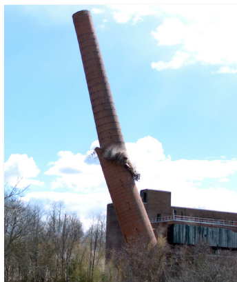
Razing Building No. 29.1 - Power Plant Smoke Stack
