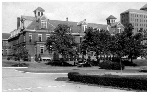
Building C - Patient Facilities
