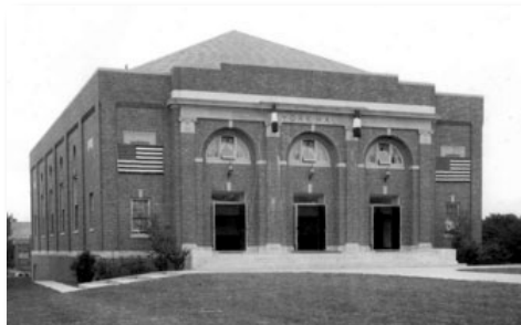
Building No. 80 - York Hall
